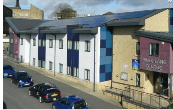
2 28kWp Solar Array at Park Lane Centre
