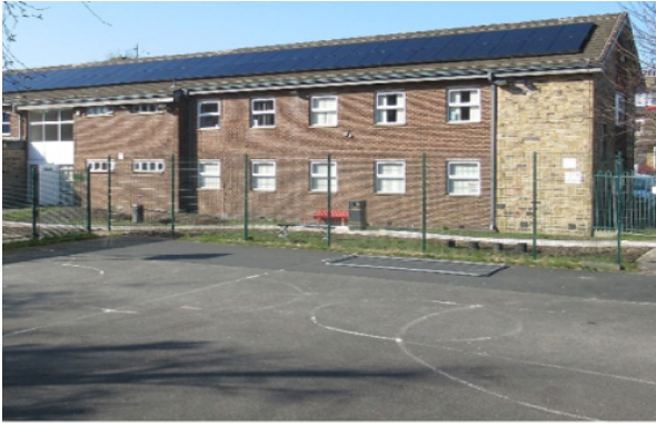
1 30kWp Solar Array at Mayfield Centre
